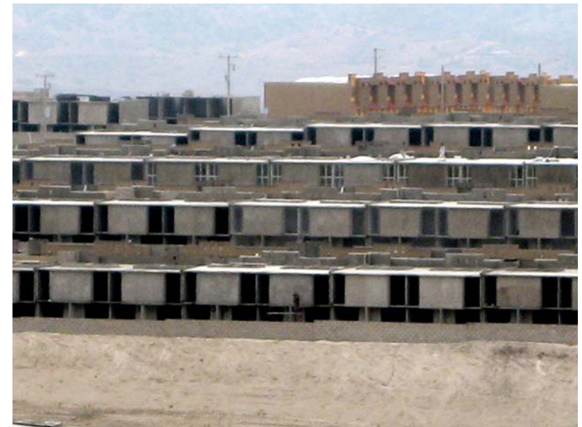
Fig. 4: “Pigeon houses” being built around manufacturing plants near Tijuana, Mexico.
